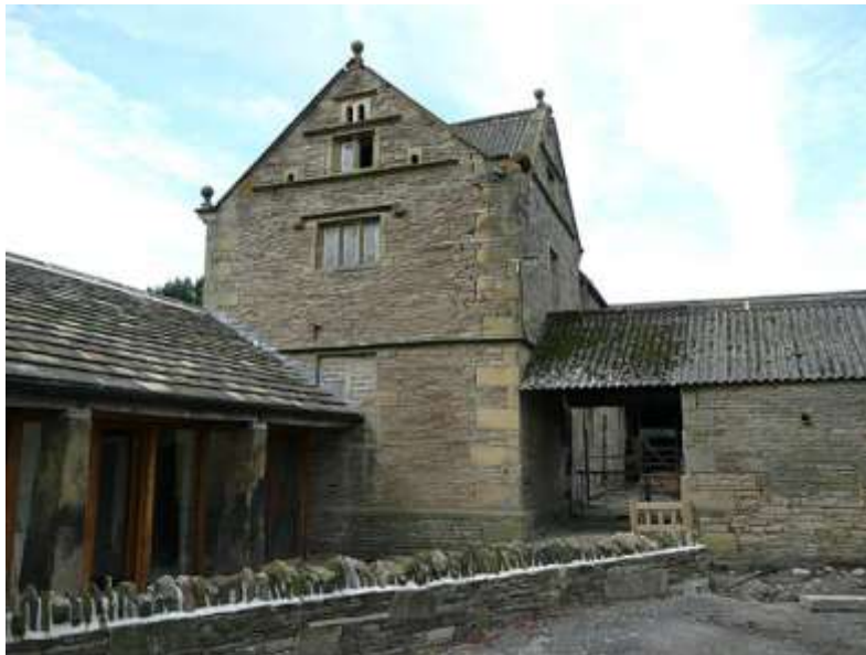
Courtyard buildings, Gunthwaite Hall
